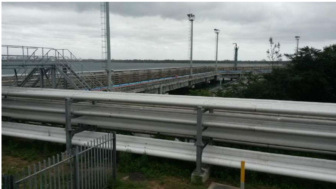
Figure 3-14: View of Berth 208 and proposed Berth 207 from control room
