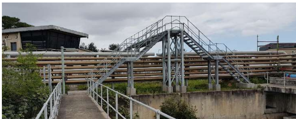
Figure 3-12: Access Walkway over Pipe Rack
